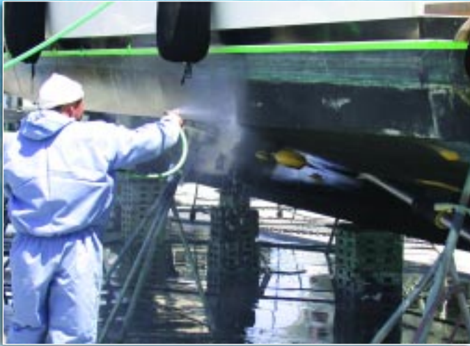
Hydro-Washing at Boat Repair Yard
