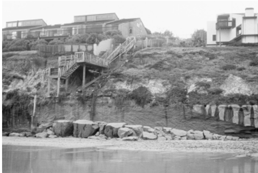
Homes built on actively eroding bluffs in San Diego County are no longer fully supported from beneath, making them vulnerable to earthquakes and landslides. Photo: California Sea Grant archives.
