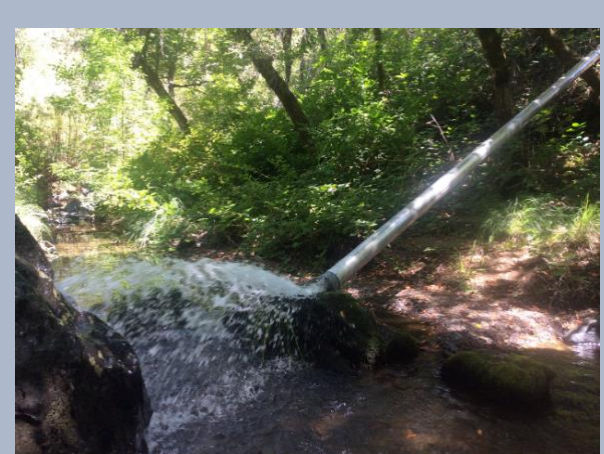
Augmentation pipeline release at 290 gallons per minute.
