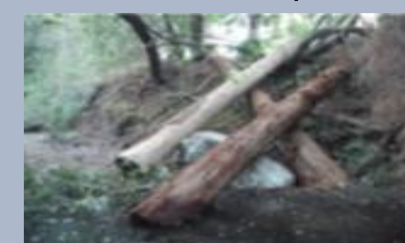
Large Woody Debris installed in Porter Creek by Sonoma Resource Conservation District
