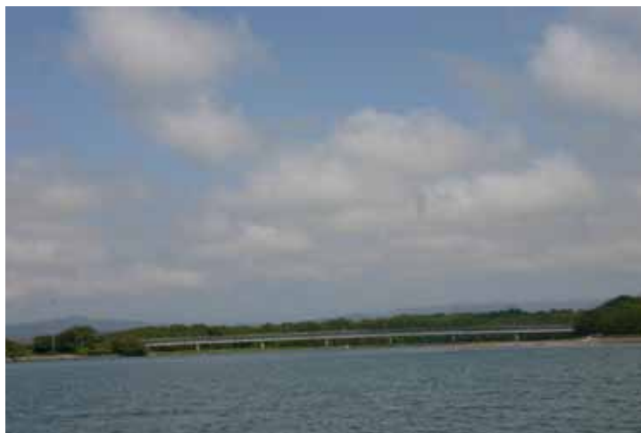
Open water at Cock Robin Island bridge
