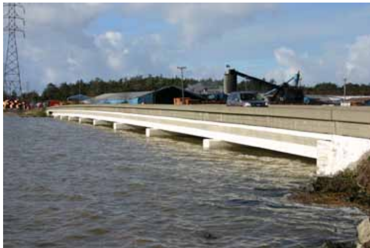
Highway 255 bridge at Mad River Slough
