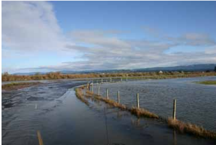
Mad River Slough flooding the road and adjacent pastures.
