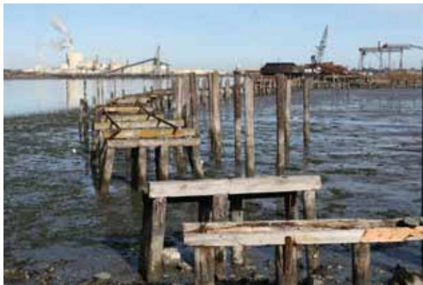
Many eelgrass beds along deep channels in Humboldt Bay have derelict pilings treated by creosote
