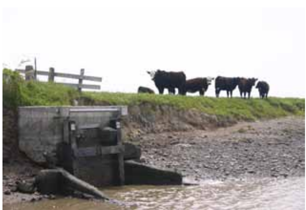
Levee without hardening
