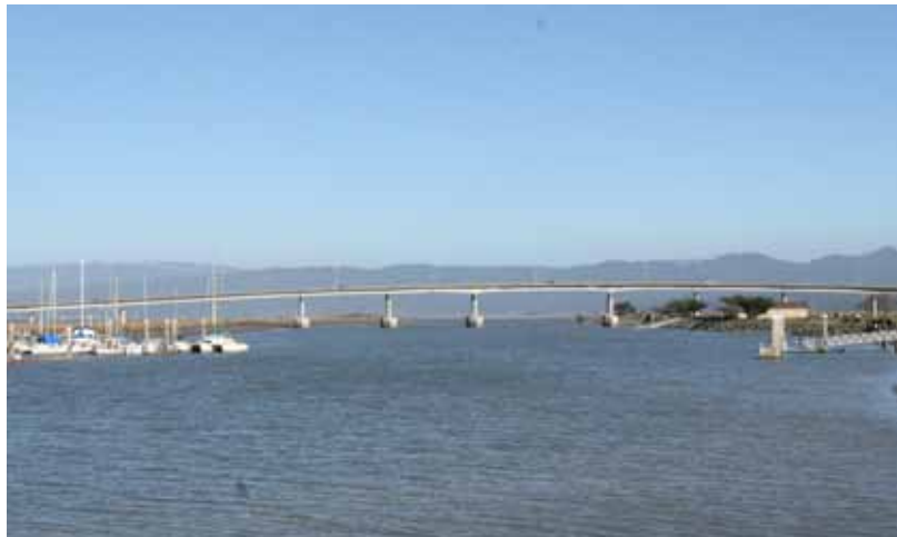
Open water near the Samoa Bridge
