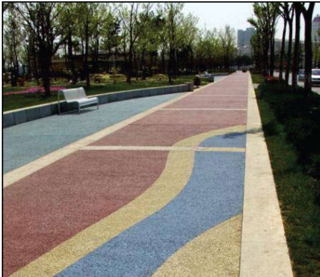
Pervious concrete can be installed in a wide range of colors to create exciting designs.
