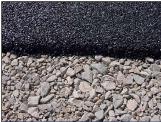
Close up of porous asphalt being installed over open-graded aggregate.
