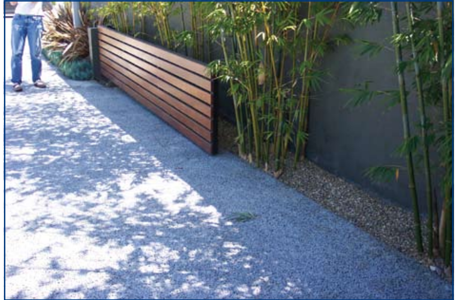
David Hertz Studio, an architectural firm in Santa Monica, has installed a permeable pavement parking lot, demonstrating its commitment to green building.
