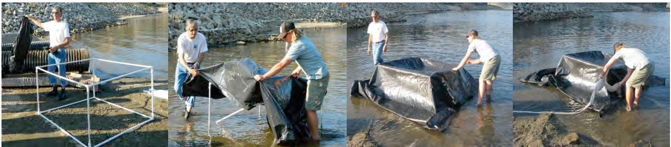
Figure 3-1. Tarping demonstration by Dr. Lars Anderson and Dan Daft at El Capitan Reservoir in San Diego County, CA. This series of pictures shows building a frame from PVC pipe to provide structure for tarps (used to cover large rocks or objects), rolling the tarp over the frame and then securing the tarp to the lake bottom with sand bags. Photo Credit: Jodi Cassell and Marsha Gear
