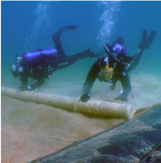
Figure 3-2. Divers rolling out mats made from aspen shavings (see “Success Story”). Photo Credit: Jim Brockett, Tahoe Resource Conservation District
