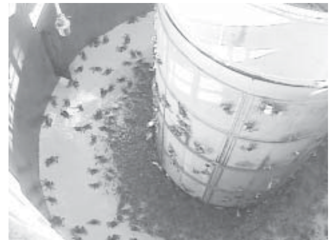
Hoads of mitten crabs clog a fish salvage system, requiring workers to drain the tank. Photo: U.S. Bureau of Reclamation
