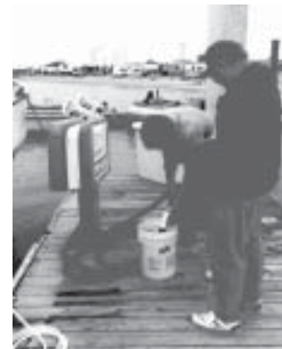
A sewage-pump-out station being checked for efficiency. Waste pumped from boats goes into the local sewage treatment system.
