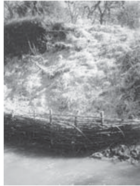
Boulder weir constructed to channel stream energy, enhance coho salmon habitat and reduce erosion.
