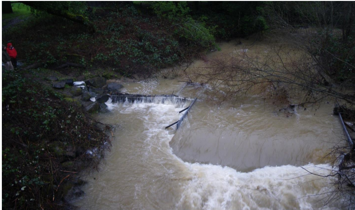
Figure 42. Mill Creek adult trap in high flow conditions when fish are able to swim around and over the trap.
