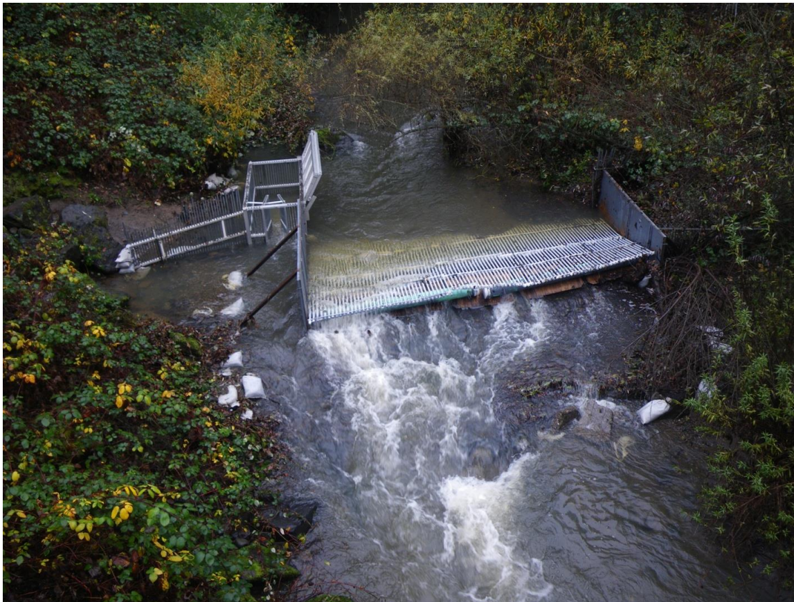
Figure 33. Mill Creek resistance board weir and trap, December, 2010.
