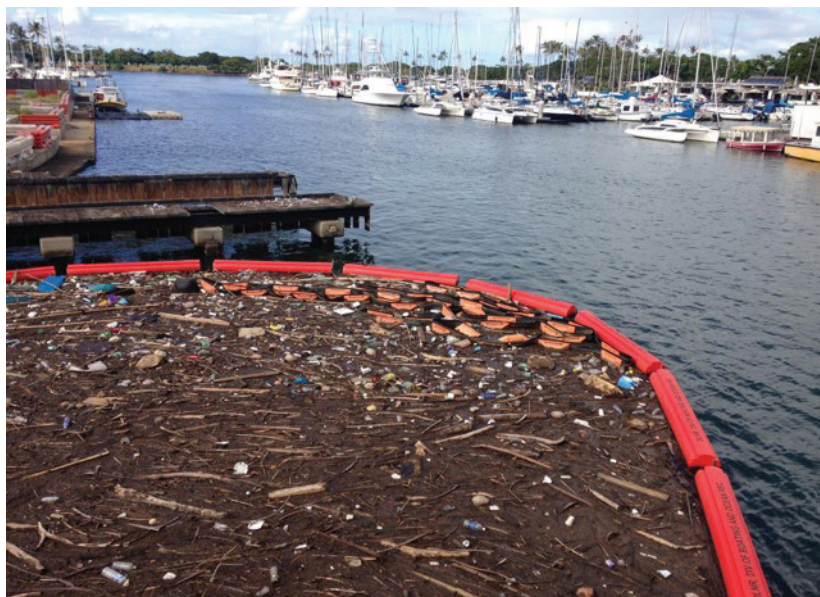
FIGURE 7.2 A debris retention boom at the Ala Wai Boat Harbor, O'ahu, Hawai'i preventing upstream debris transported via the Ala Wai Canal from entering coastal waters. Image courtesy of Mary J. Donohue.
