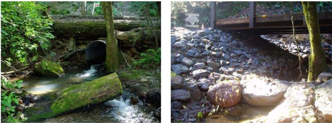
Figure 18. Wine Creek flowing under Koch Road (before and after crossing modification)
