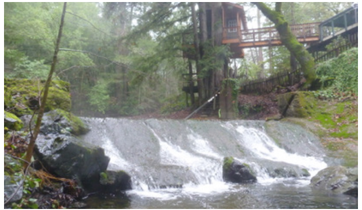
Historic flashboard dam on Mill Creek, prior to remediation.
