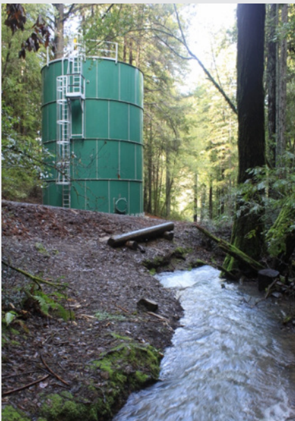
Water storage tanks were installed to capture spring water in place of a direction diversion from Dutch Bill Creek.
