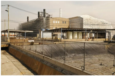
Portions of the shuttered Exide Technologies facility in Vernon, about 5 miles from downtown Los Angeles, are wrapped in white plastic to prevent the release of lead and other harmful pollutants. (A1 Seb) / Los Angeles Times
