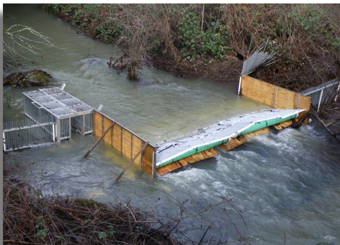
The adult trap, with a resistance board weir, is able to ride out high flows and debris with minimal damage while providing a low-flow holding structure.
