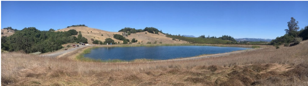
Figure 2. Existing approximate 250-acre foot storage pond on the E & J Gallo MacMurray Ranch property.
