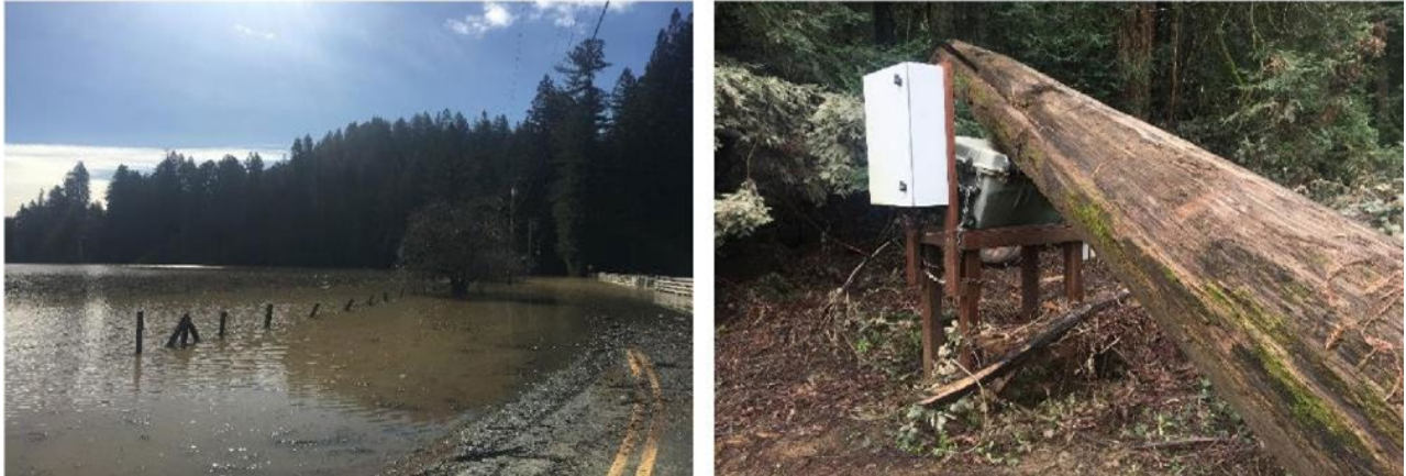
Figure 37. Westside Road during flood event and subsequent damage to PIT tag transceiver.
