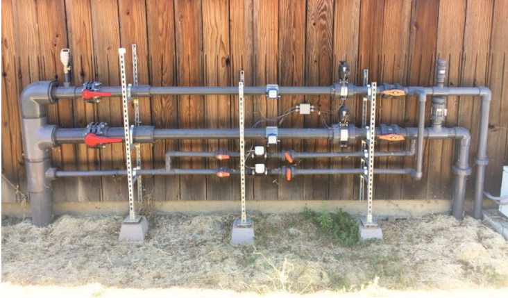
Figure 4. Valve and meter system (pictured left) and the system controller (pictured right) for the Porter Creek flow augmentation system.
