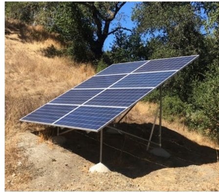
Figure 5. Pictured left, existing pumphouse located below the storage pond that was used for housing system control infrastructure with the constructed photo-voltaic array that provides power to the controller and valve actuator in the background (also pictured right).
