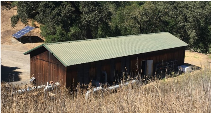
Figure 5. Pictured left, existing pumphouse located below the storage pond that was used for housing system control infrastructure with the constructed photo-voltaic array that provides power to the controller and valve actuator in the background (also pictured right).
