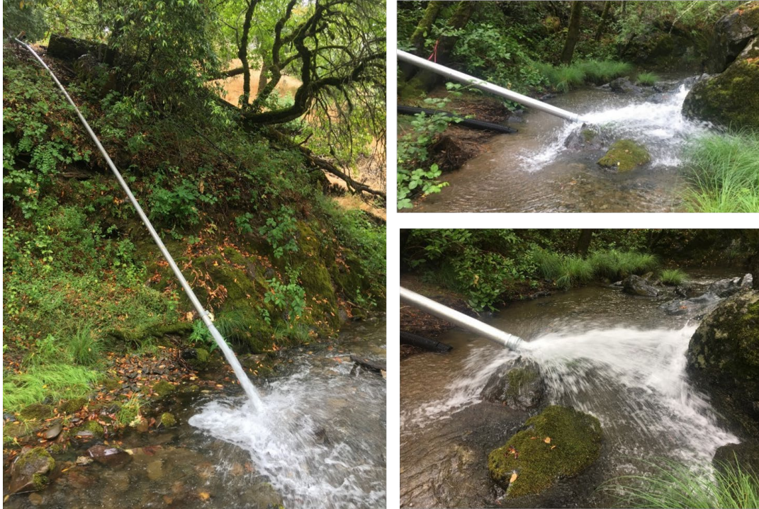
Figure 6. Water releases from the E & J Gallo MacMurray Ranch storage pond into Porter Creek. Pictured left, removable section of aluminum pipe at the upper release site. Pictured right (top and bottom), removable section of aluminum pipe at the lower release site.
