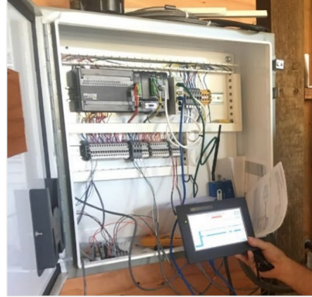
Figure 4. Valve and meter system (pictured left) and the system controller (pictured right) for the Porter Creek flow augmentation system.
