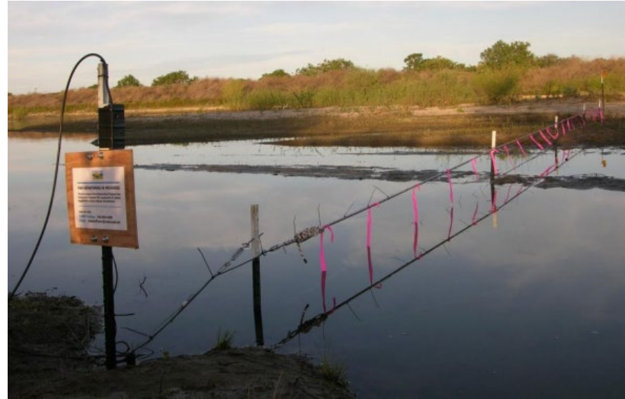
HDX swim through PIT antenna on the San Joaquin River (image: Bureau of Reclamation)
